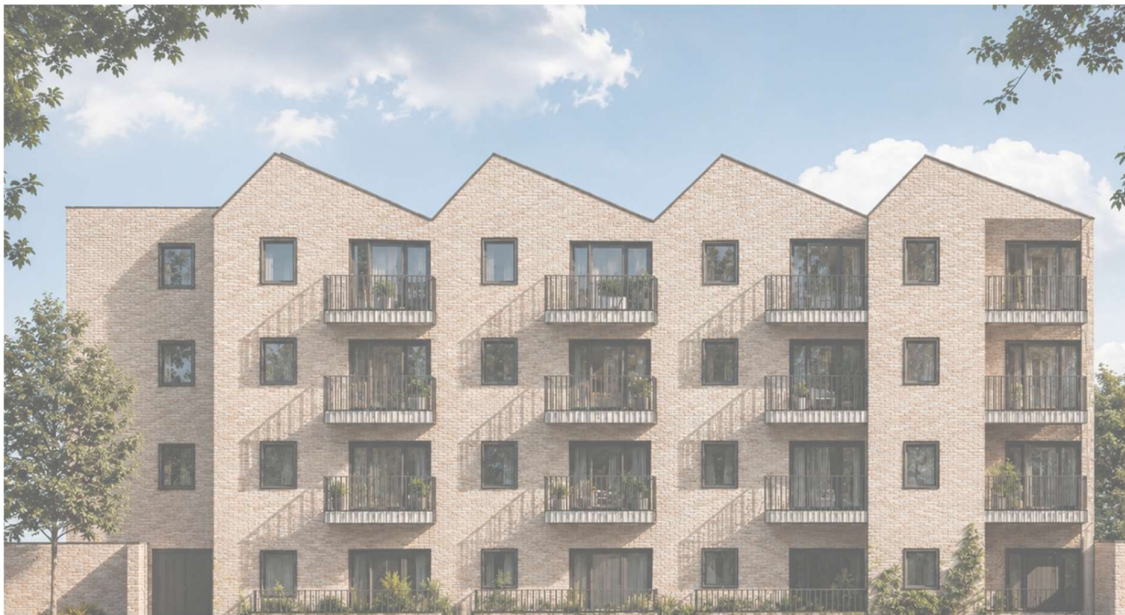
16no Units at form Central Garage Site, Parnell Road, Bray
